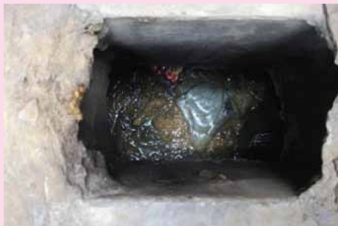
Solid waste that has been disposed of in a pit latrine (Photo: Belen Torondel/LSHTM)
