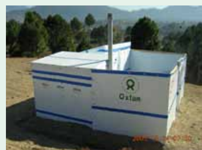
Screened latrine and bathing unit
