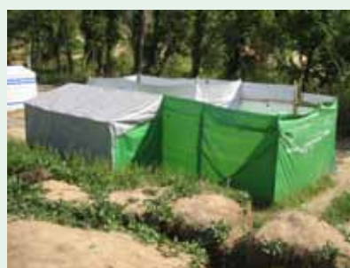
Screened latrine and bathing unit with internal menstrual slab and raised sides for additional privacy
