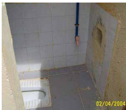
Disposal shoot inside the latrine
